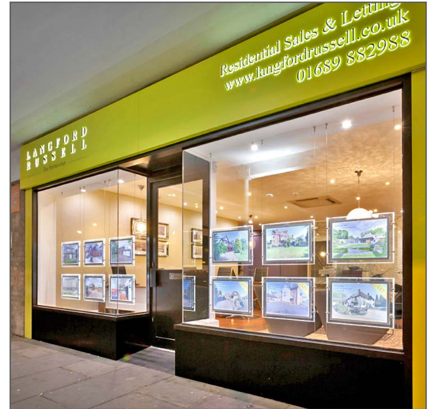
Internally LED illuminated aluminium sign tray. All text fret cut with acrylic pushed through from the rear (10mm). Individual letters faced with vinyl to create a halo (glow) effect. Includes LED window displays.
