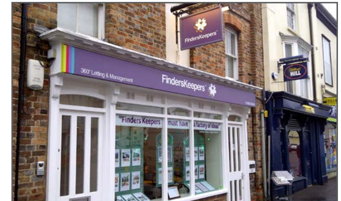
Aluminium composite sign tray with digitally printed vinyl graphics. Finished off with an illuminated projecting sign.
