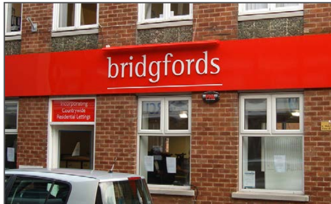
Aluminium composite sign tray with 5mm white acrylic stand off lettering and illuminated parabeam (strip) lighting.
